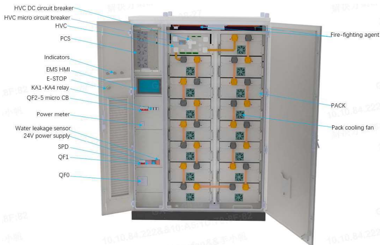
Figure 2.6-2 Cabinet Interior Structure Diagram
